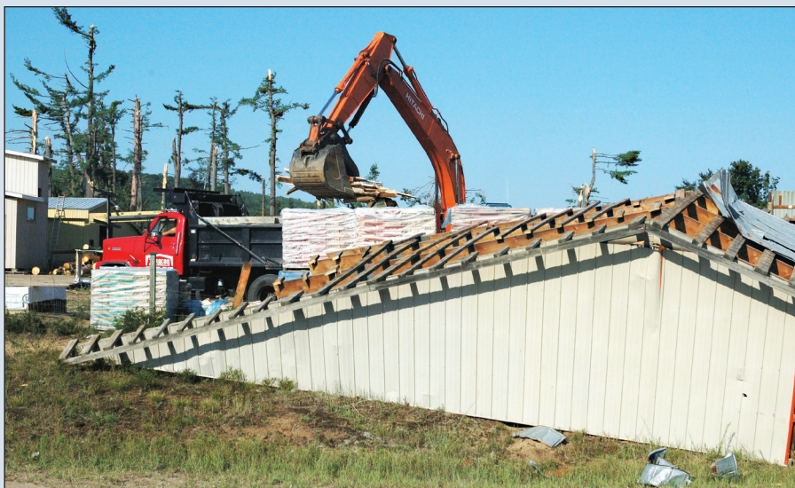
Crews picking up the pieces after Home Hardware's roof was ripped from the building and thrown onto the highway. Photo Kent Waddington Photography
