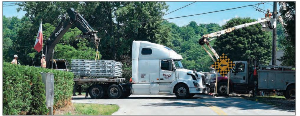
Construction crews have begun preparing the north and south approaches for the installation of a modular bridge that will temporarily replace the collapsed Imperial Road Bridge to Port Bruce, Elgin County, which is responsible for both the collapsed and temporary bridges, expects the new crossing over Catfish Creek to be ready for traffic in August. (AE/Rob Perry)
